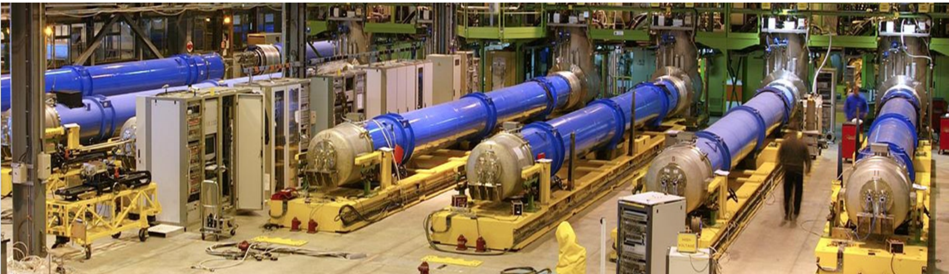
Sm18 Hall - Test Banches
